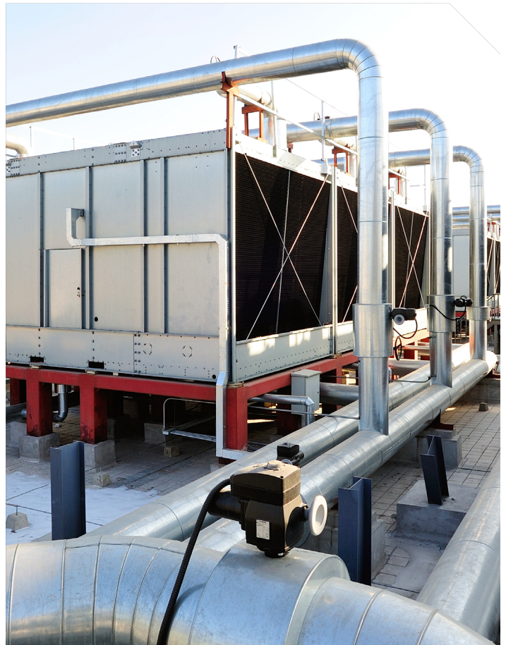
Sets of cooling towers in data center building. Image credit: Adobe
