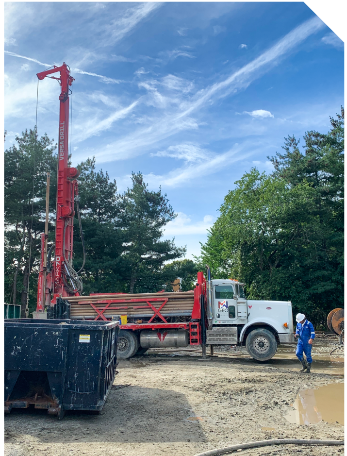
A geothermal borehole drilling rig.
