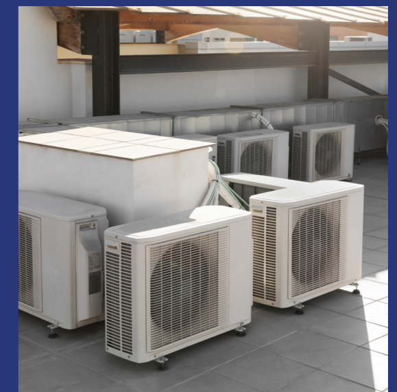
Packaged Rooftop Unit (RTU)
