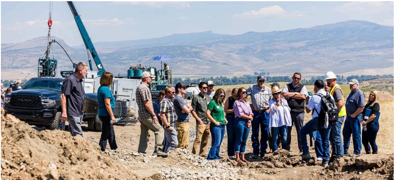
Derek Kobe of Green Built Construction and Fernando Aguilera of Bedrock Energy lead a tour group at the thermal energy network construction site. Photo credit: Brooke Ashlee Photography.
