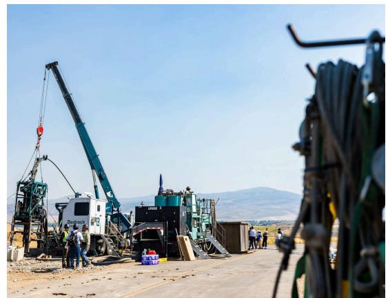
Bedrock Energy began drilling Phase 1 in 2025. Photo credit: Brooke Ashlee Photography.
